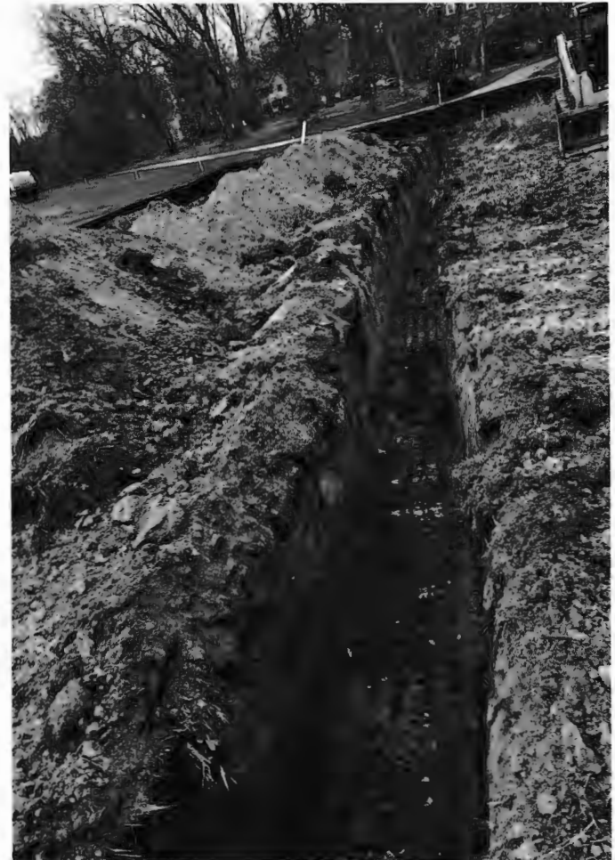
Septic tank to d-box to trenches
