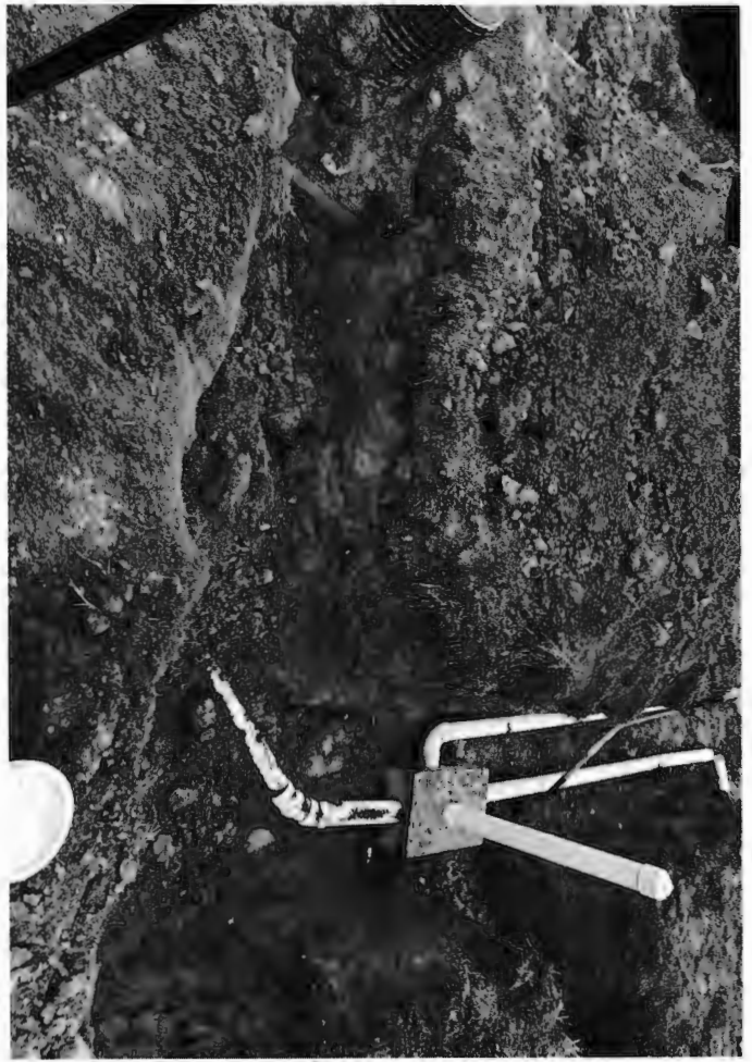
Septic tank to d-box to trenches
