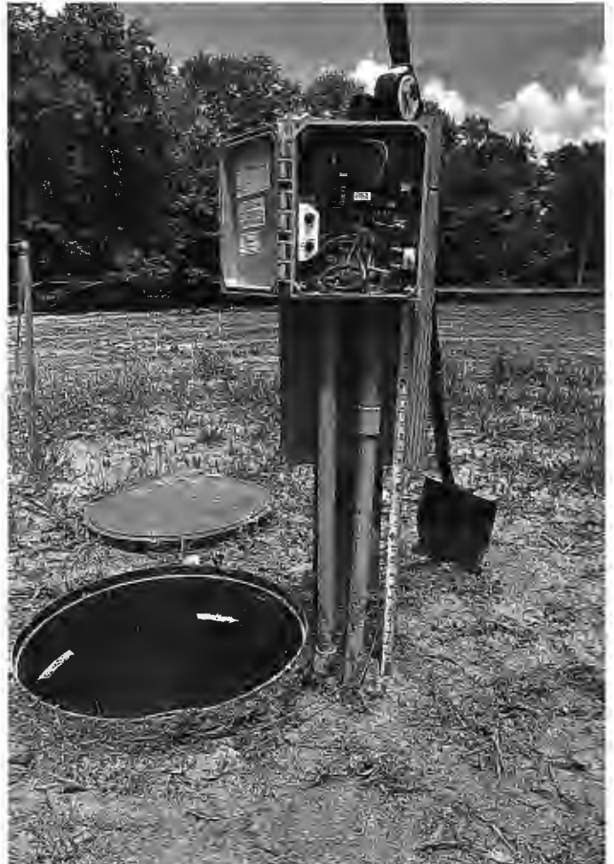
7/11/25 2nd inspection. Control panel @ 30" above grade
