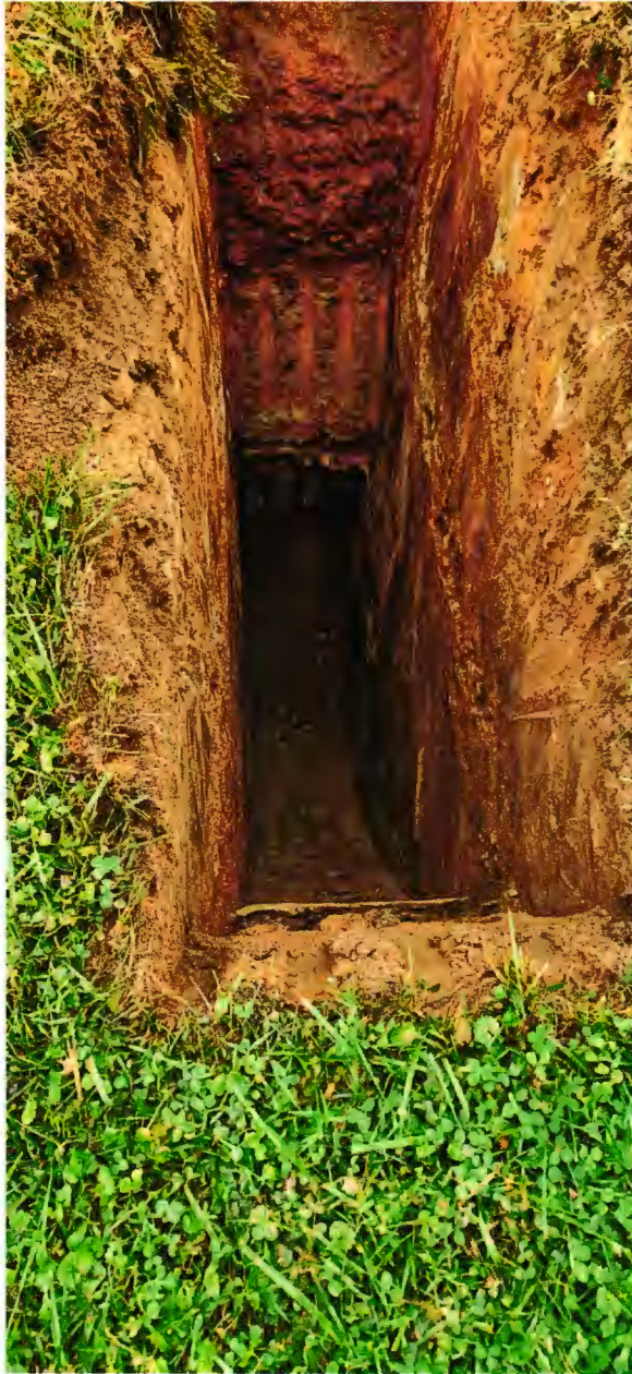
Perc test hole dug between last trench and driveway to 14 feet.
