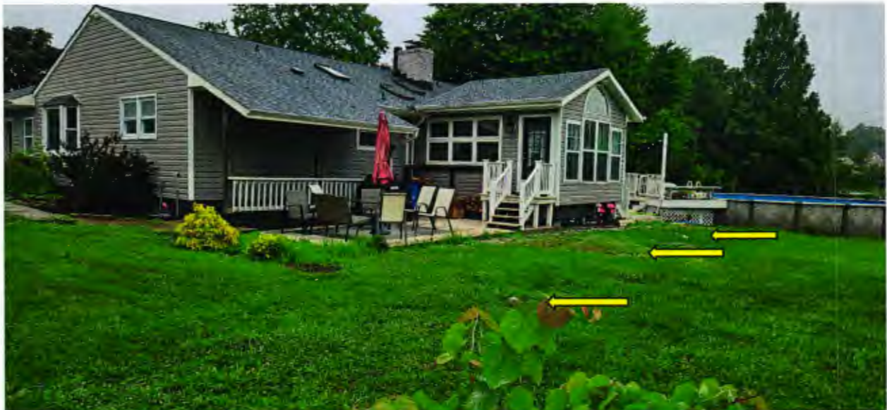
Cleanouts over tank, and both d-boxes.
