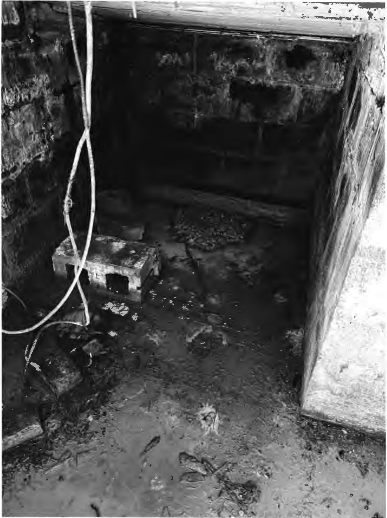
6/26/2025 - Abandoned dug well inside House (P)
