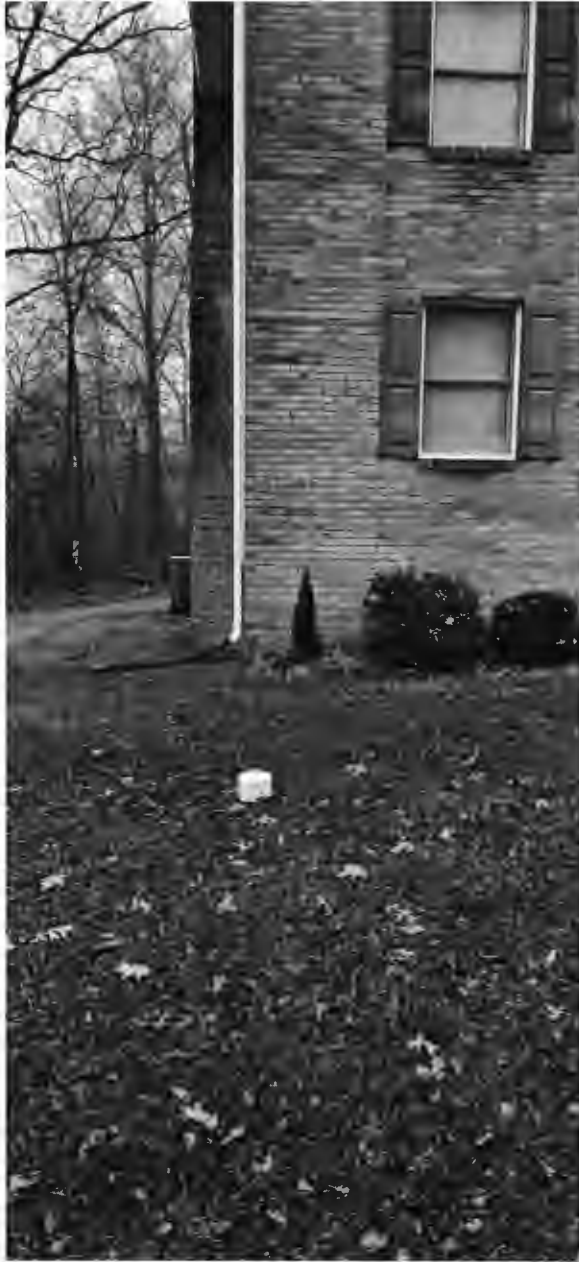
Septic Tank Cleanout in front
