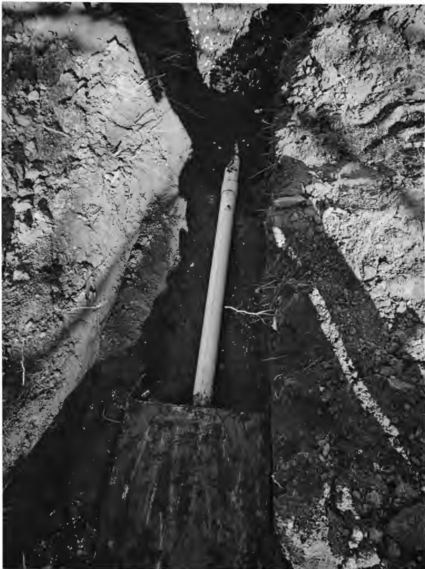
3/27/25 Remains 4' of pipe installed. (M3)
