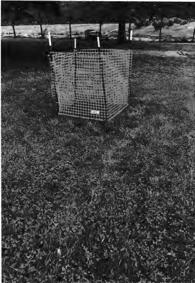
Septic tank clean out
