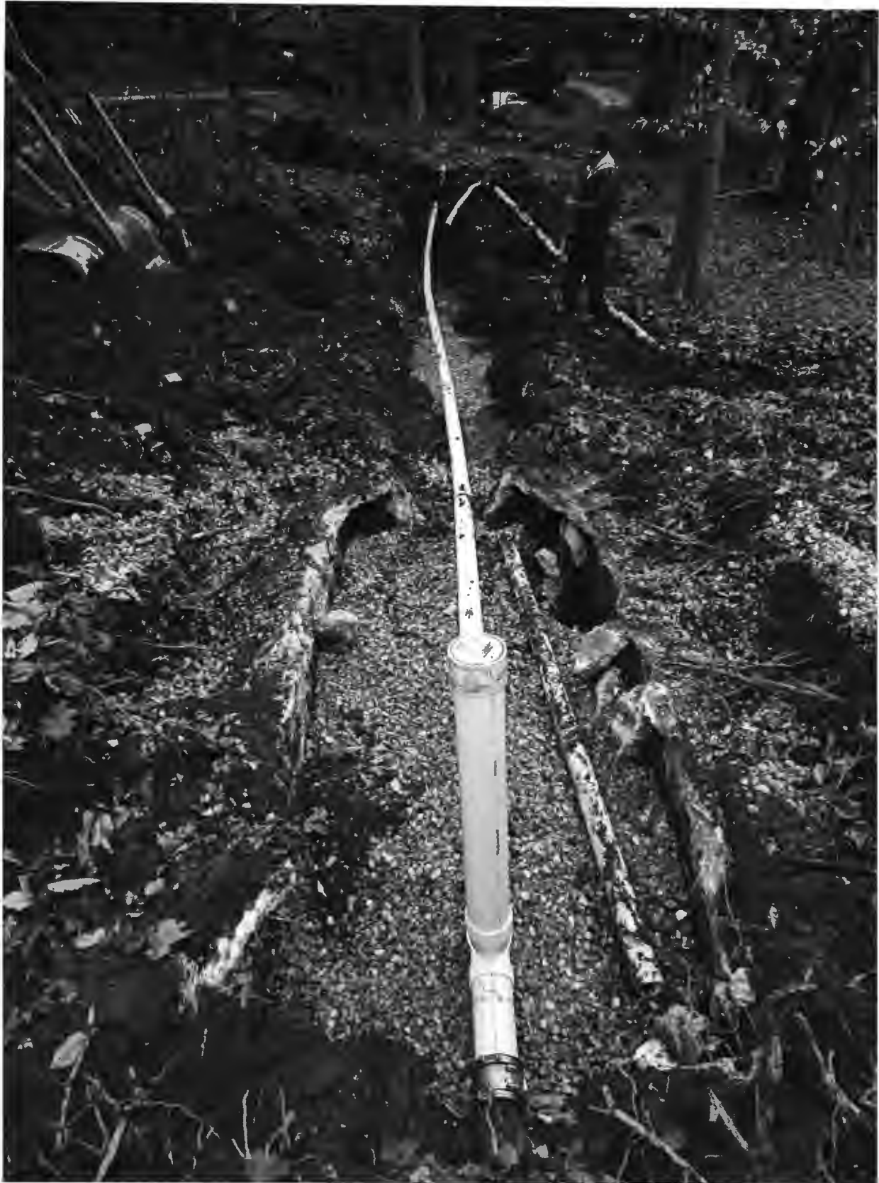
12/13/2024- Rec'd Pics of Finished install. 68' of 4" SCHD 40 PVC installed. SP
