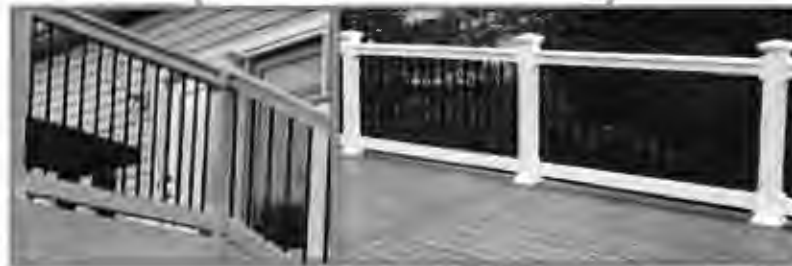
Example of white vinyl railing that will be used throughout the deck as well as the stairs. The vinyl railing will be either 36" or 42" (based on final design preference) and will contain black aluminum balusters, as shown.
