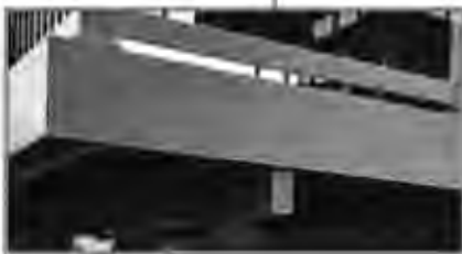
Example of white PVC trim board that will accent the outside of the deck and stair stringers
