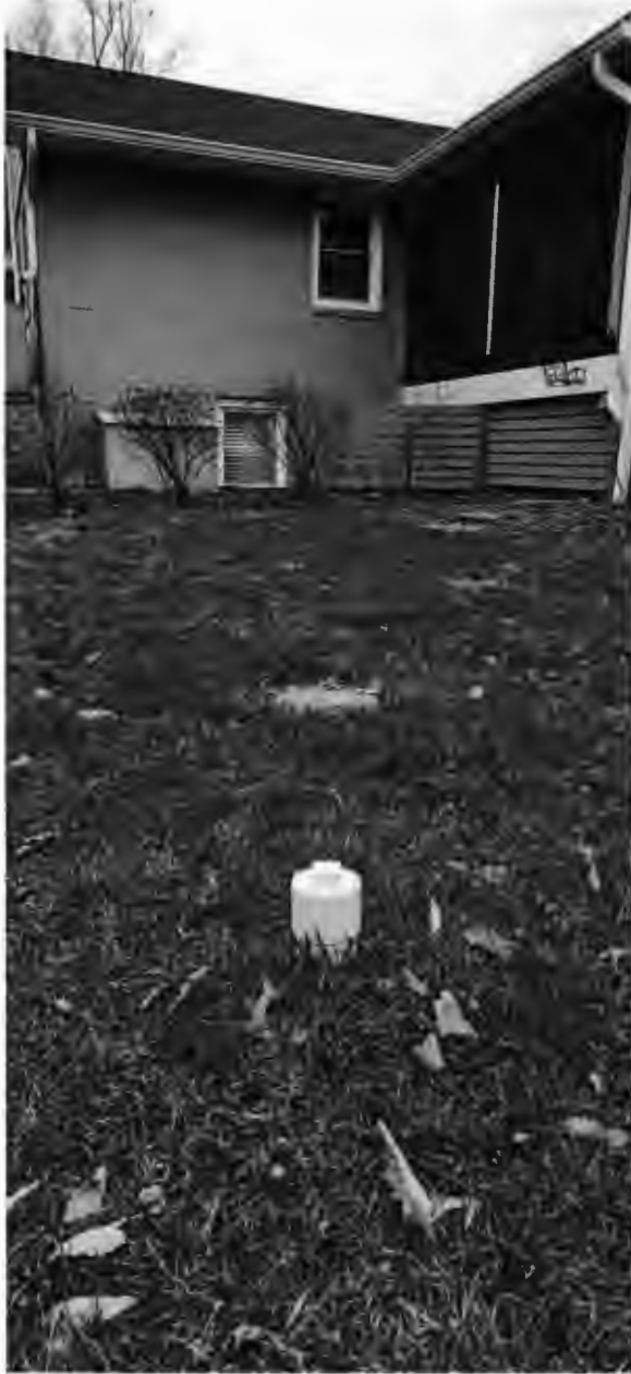
Septic Tank Cleanout
