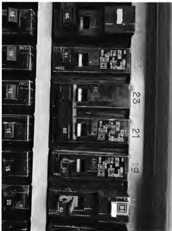
3/15/2024 - 2 Breakers installed for septic p & A system
