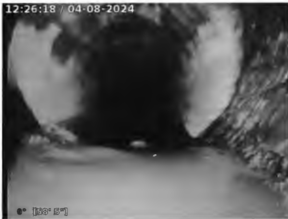
Transition back to PVC and start of third belly.
