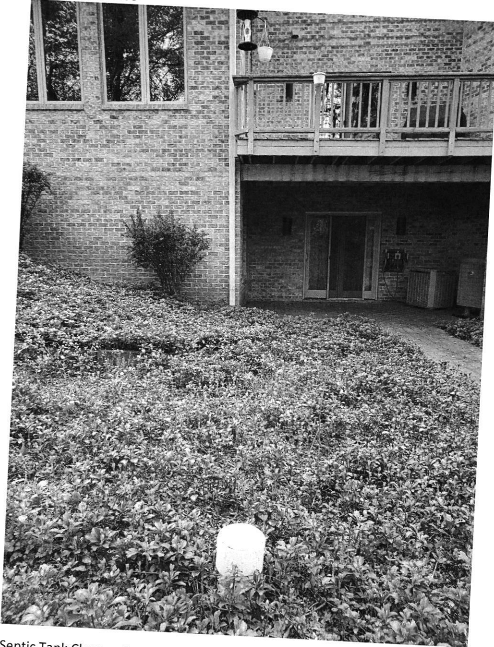
Septic Tank Clean-out
