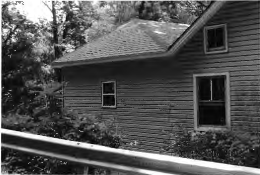
Second floor addition from road, left side
