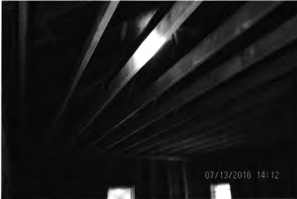
Second floor --ceiling/roof framing
