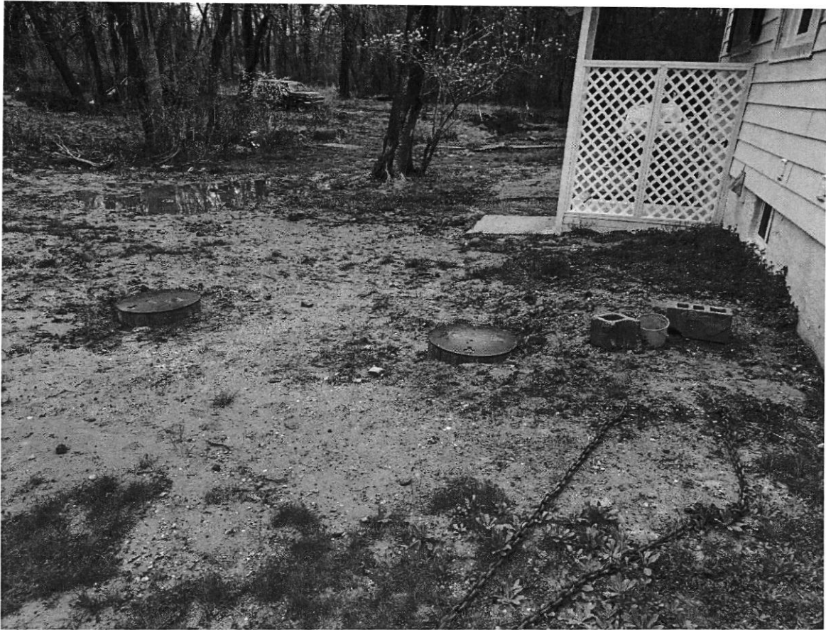
Photo along the proposed house connection for 10416 Guilford Road. Note ex. holding tank.
