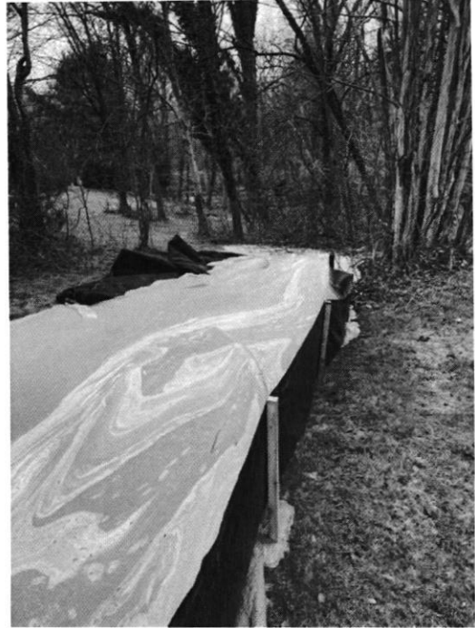
10161 Maxine Street, Ellicott City, MD. 21042 – sediment and foam from drilling activities running into a stream (MD State Waters) 1/11/2023
