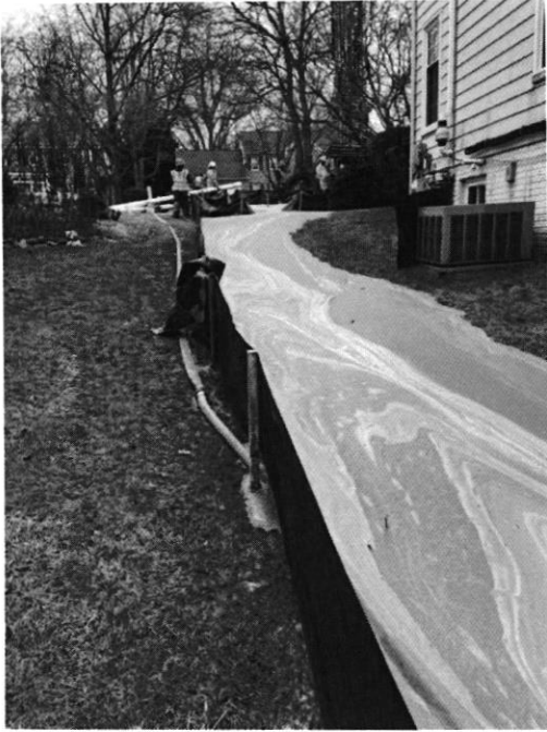
10161 Maxine Street, Ellicott City, MD. 21042 – sediment and foam from drilling activities running into a stream (MD State Waters) 1/11/2023
