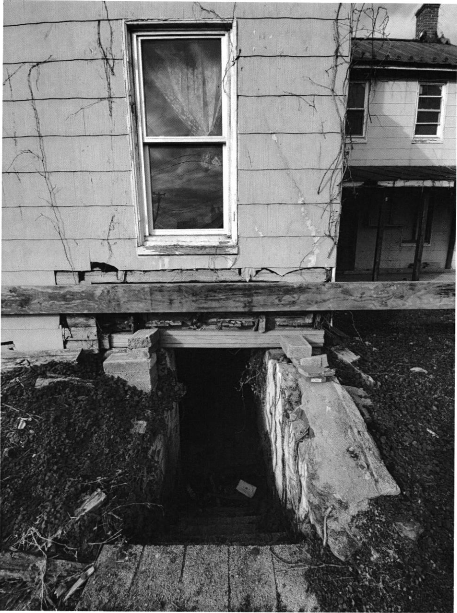
Site Inspection – 12.15.21 15904 Frederick Road
