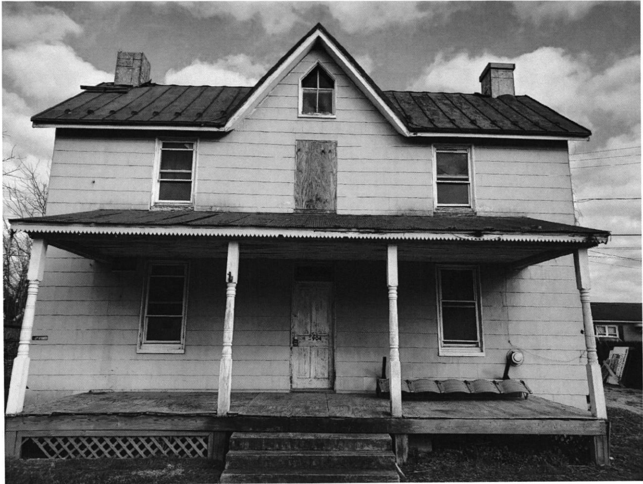
Site Inspection – 12.15.21 15904 Frederick Road
