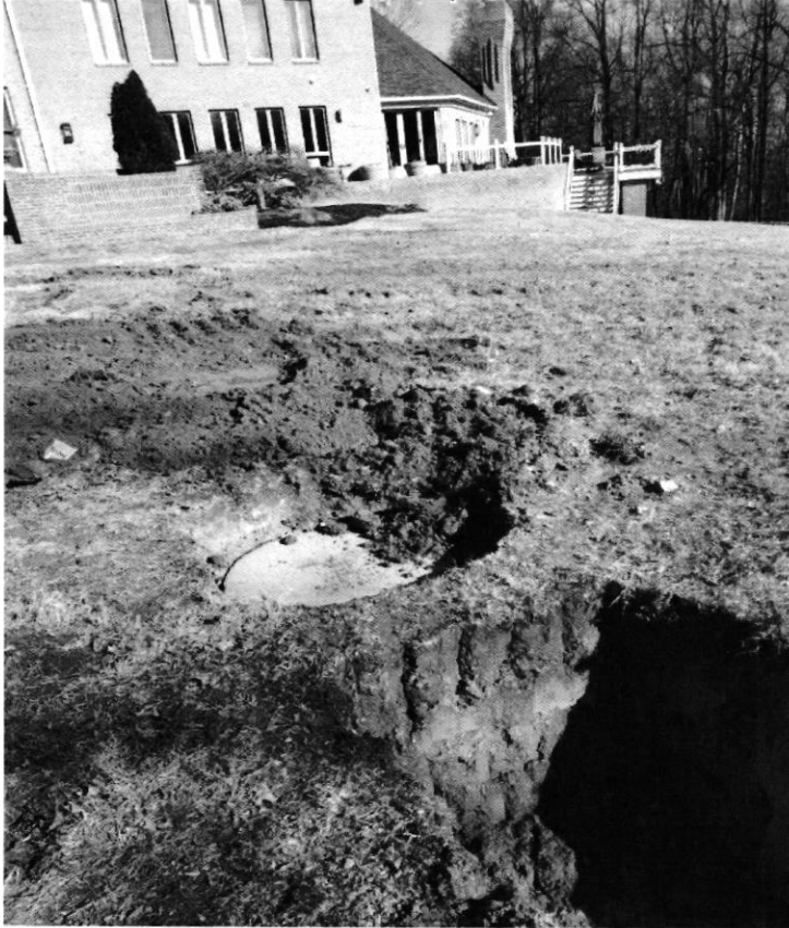
13037 Hall Shop Road – Picture of existing septic tank (aprx. 3' below grade) and Dist. Box with 4" pvc plumbing to trenches. –KMW 1/25/18
