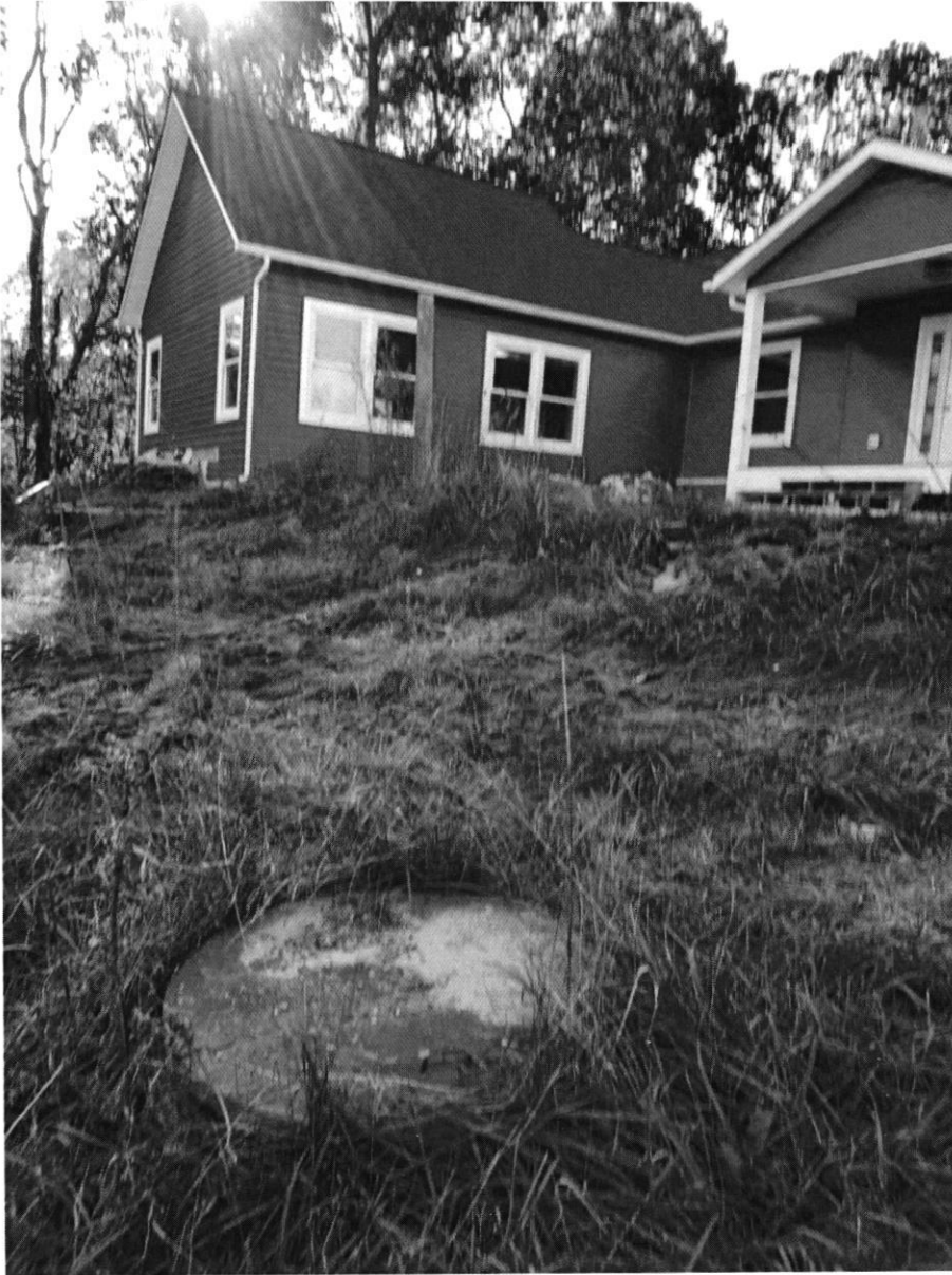
Septic Tank Cleanout
