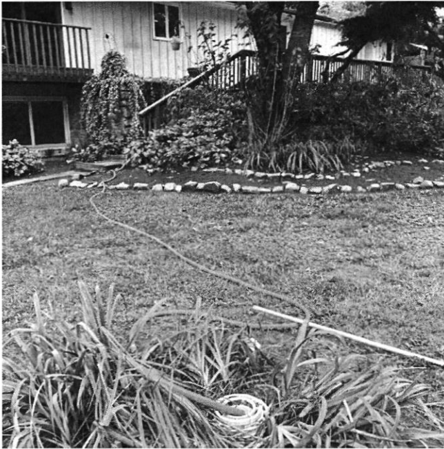
Picture 1: Showing the location of the septic tank in relation to the house.
