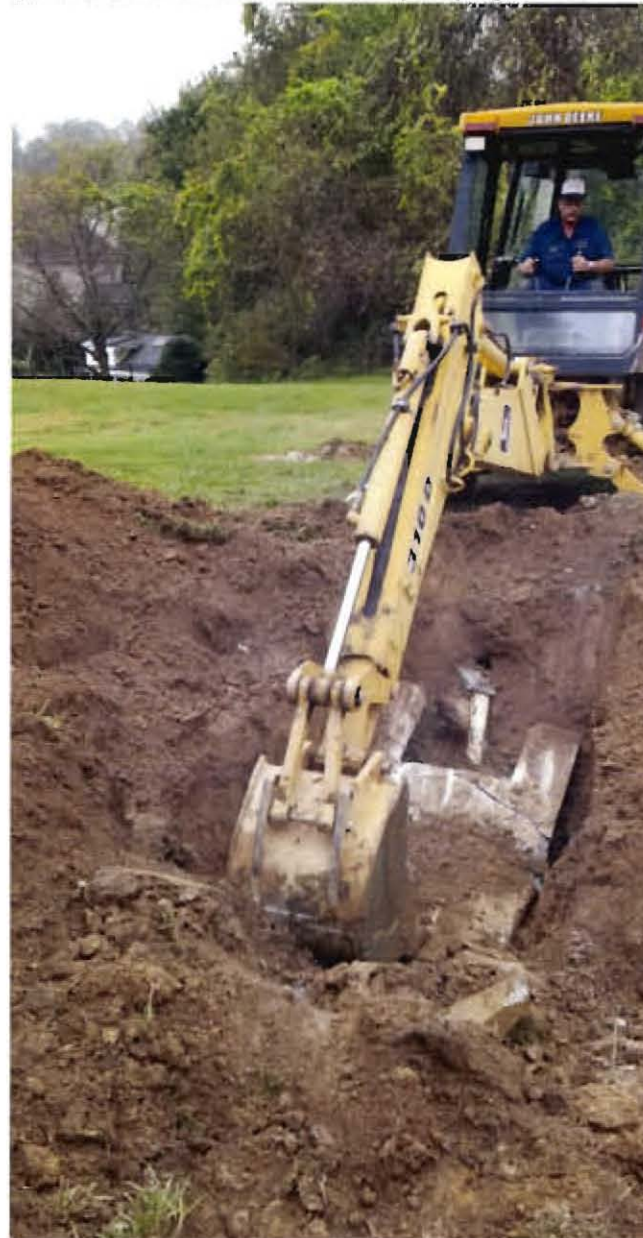
Pictures submitted by applicant on 3062 Bethany Lane Demolition request. Pictures show contractor pumping and abandoning existing septic. (10/17/2018)
