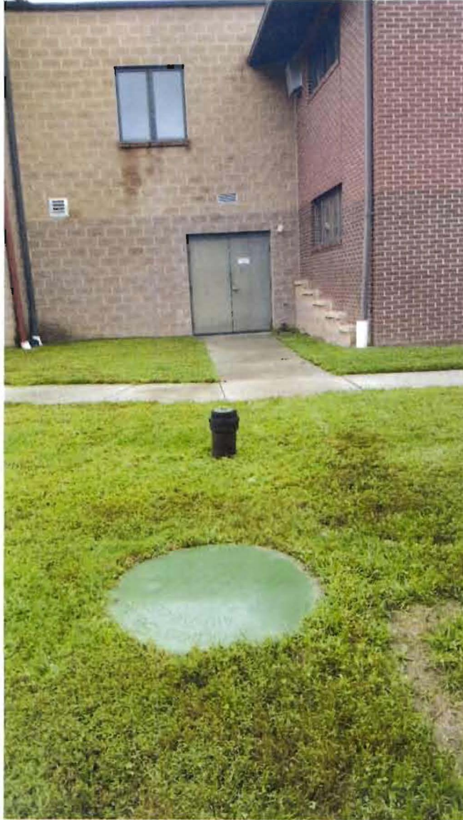
Septic tank cleanout in rear of building
