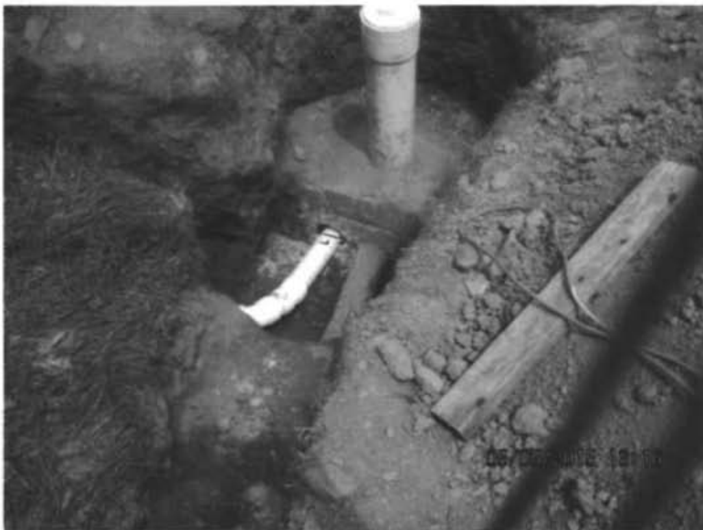
New sewer line added to septic tank
