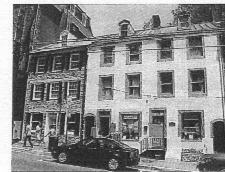
ELLICOTT CITY – masonry and siding, window surrounds, metal roof, roof dormers
