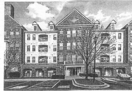
THE VILLAS OF RIVER HILL, CLARKSVILLE – brick masonry and siding composition, roof dormers, metal roofs
