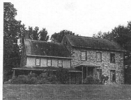
CARROLL COUNTY HOUSE – masonry and siding, window surrounds, gable roof
