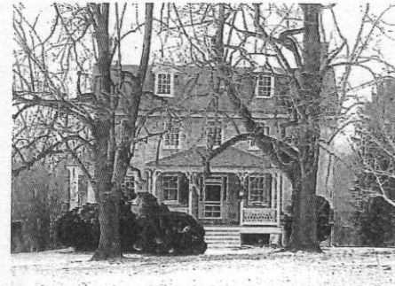
MONTROSE, CLARKSVILLE – stone masonry, red metal roof, roof dormers, hipped roof porch
