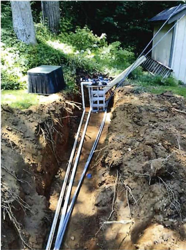
Supply, return, and check valves running to headworks
