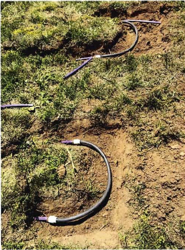
13760 Nichols Drive – installation of drip system
