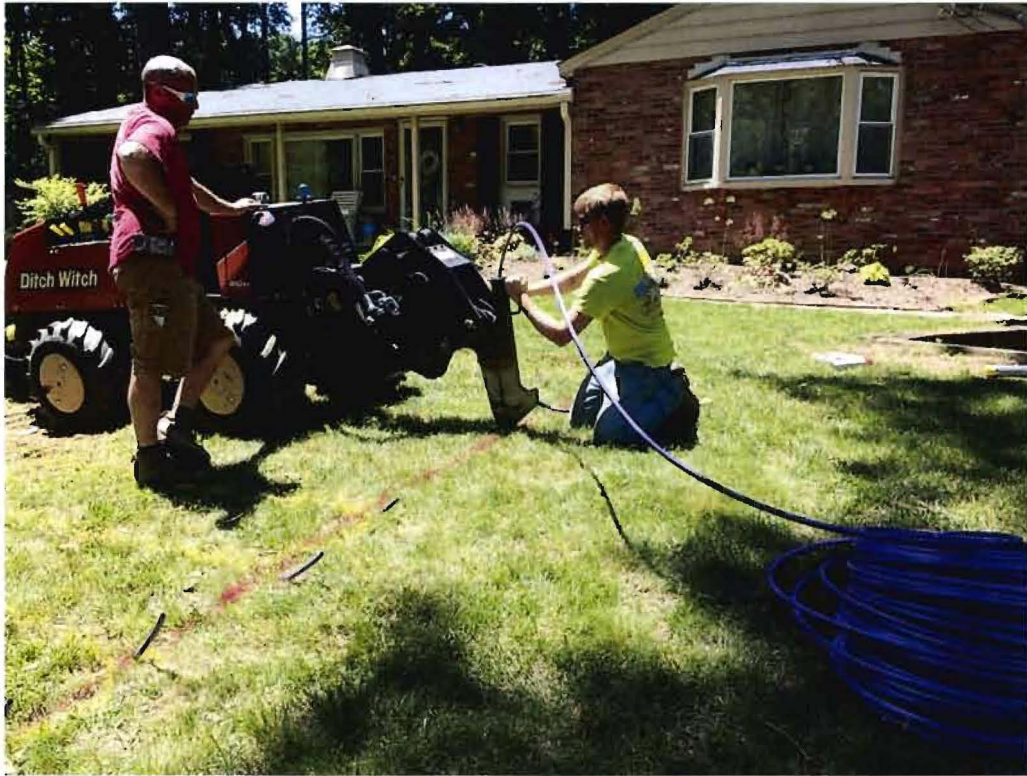
13760 Nichols Drive – installation of drip system
