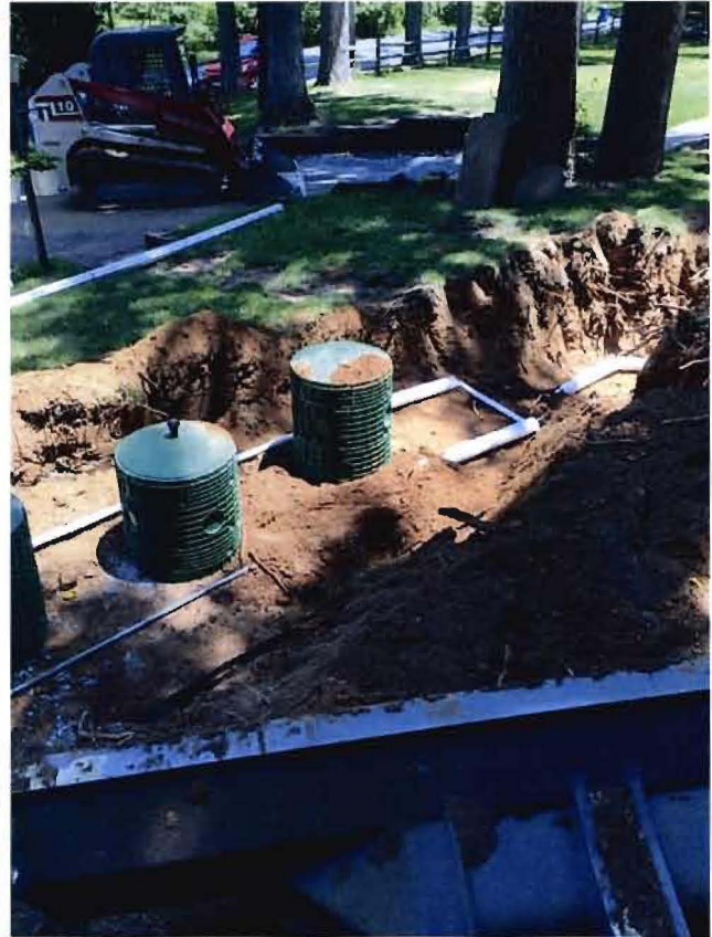
Lines sleeved running over tanks
