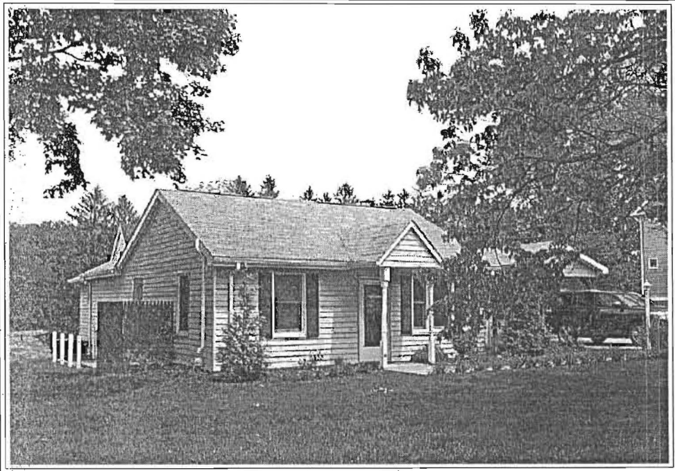
ADDITIONAL FRONT VIEW OF SUBJECT PROPERTY
