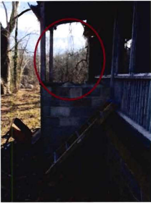
TANK #3 – TANK REMOVED
