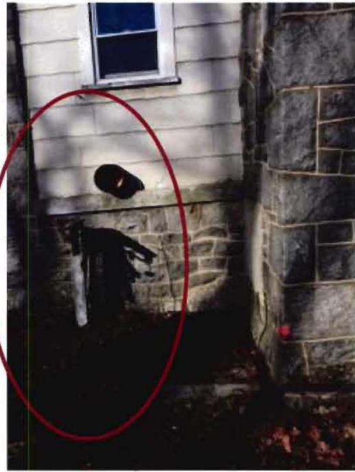
TANK #2 AFTER – VERTICAL REMOVED
