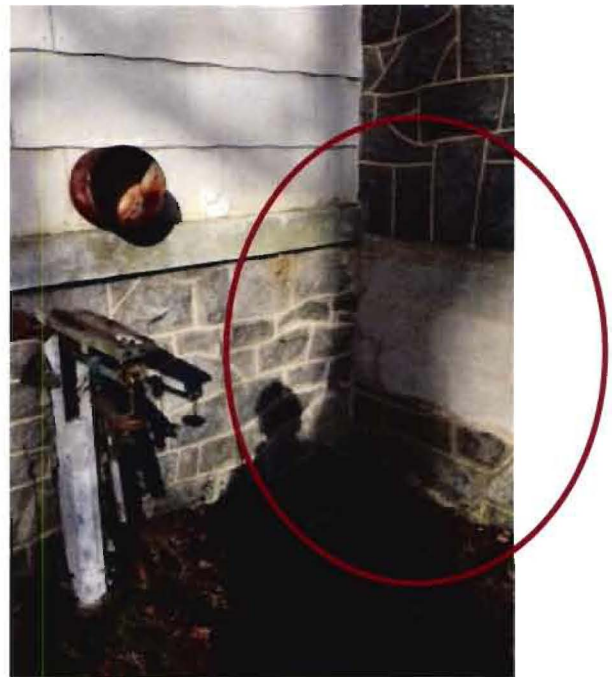
TANK #2 AFTER – TANK REMOVED
