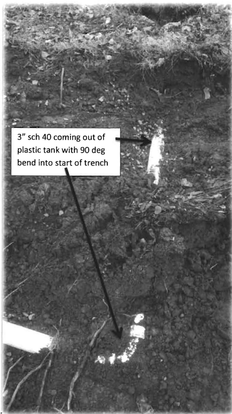
7528 Flamewood Drive – 1/30/17 Pictures of unpermitted septic sytem. Plastic Norwesco 1500g tank floated out of ground. -kmw
