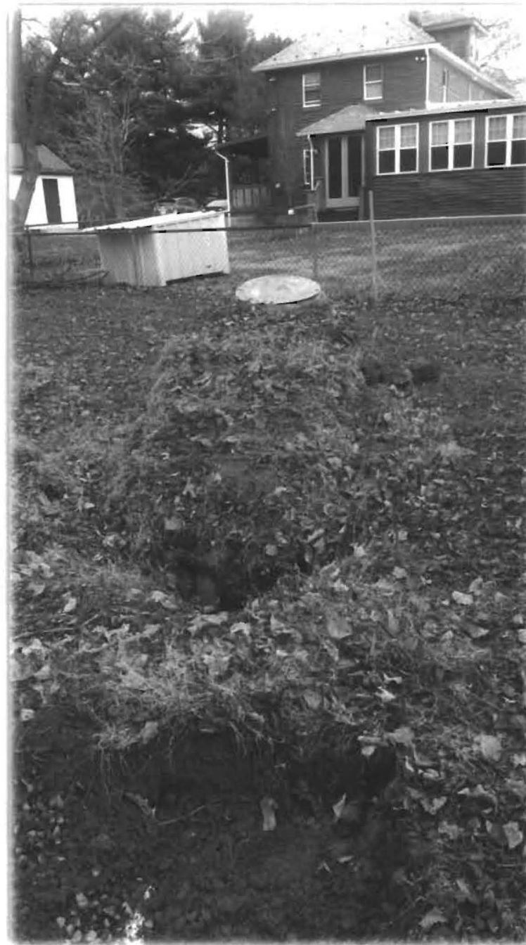
7528 Flamewood Drive – 1/30/17 Pictures of unpermitted septic sytem. Plastic Norwesco 1500g tank floated out of ground. -kmw
