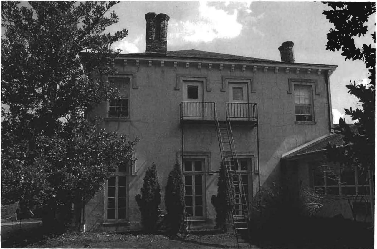
HISTORIC GLENELG MANOR — GLENELG COUNTRY SCHOOL FIRE ESCAPE NUMBER 1 - EXISTING CONDITIONS NARROW, STEEP AND UNSTABLE
