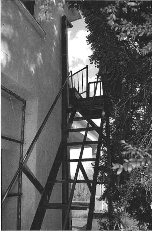
HISTORIC GLENELG MANOR — GLENELG COUNRTRY SCHOOL FIRE ESCAPE NUMBER 2 - EXISTING CONDITIONS NARROW, STEEP AND UNSTABLE
