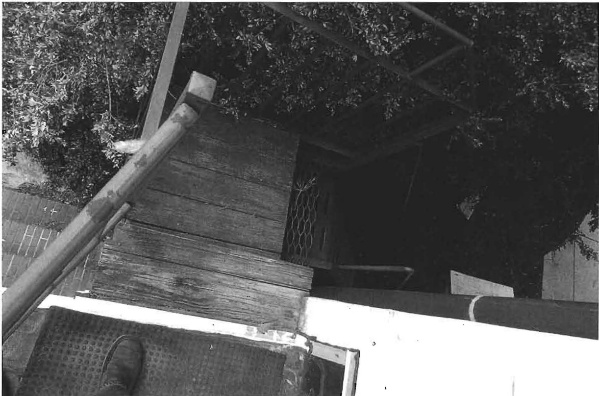
HISTORIC GLENELG MANOR — GLENELG COUNRTRY SCHOOL FIRE ESCAPE NUMBER 2 - EXISTING CONDITIONS NARROW, STEEP AND UNSTABLE
