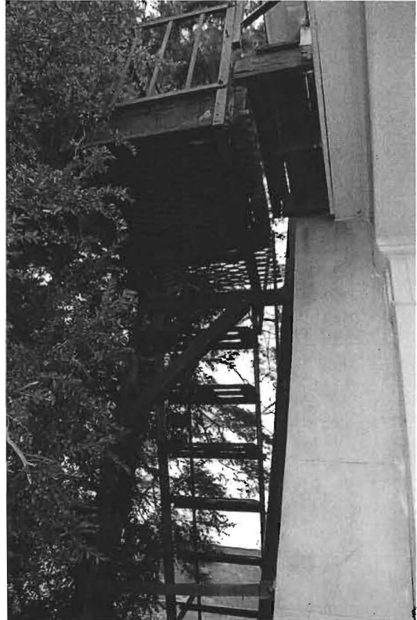
HISTORIC GLENELG MANOR — GLENELG COUNRTRY SCHOOL FIRE ESCAPE NUMBER 2 - EXISTING CONDITIONS NARROW, STEEP AND UNSTABLE
