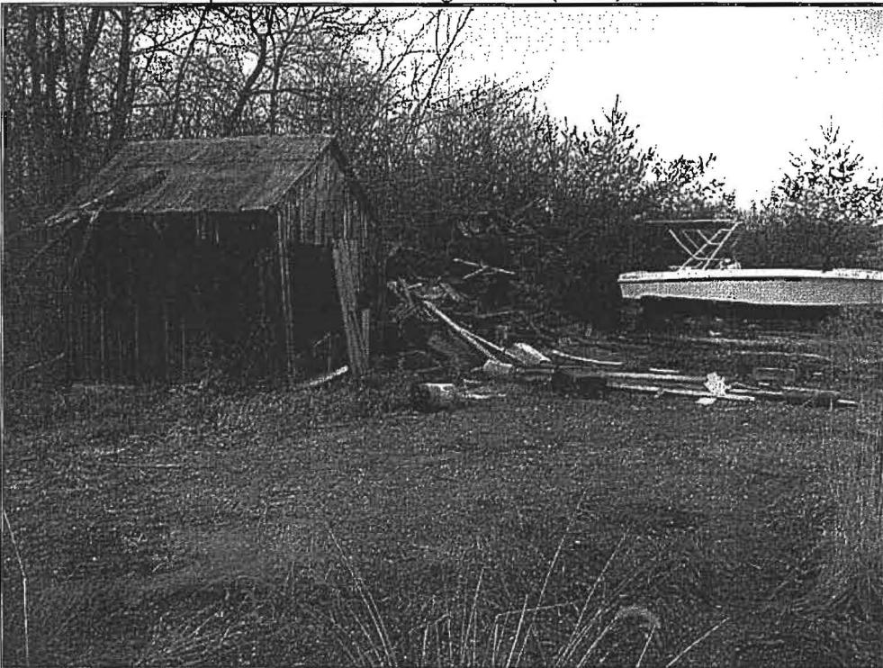
Photograph #4 - Scrap lumber, discarded tires, bricks, trash, and additional debris was observed behind and around the dwelling.
