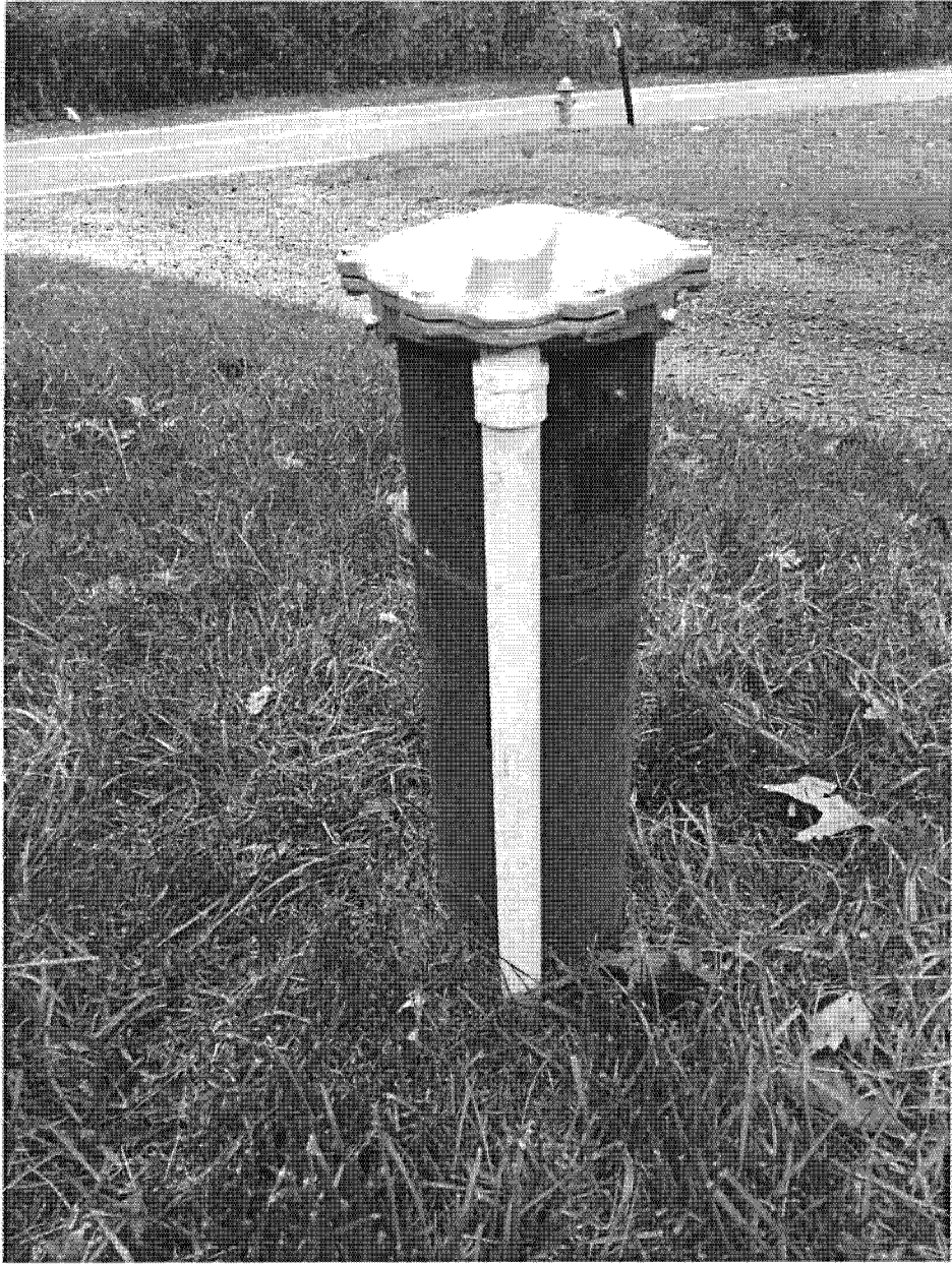
PVC line is flush with well cap.
