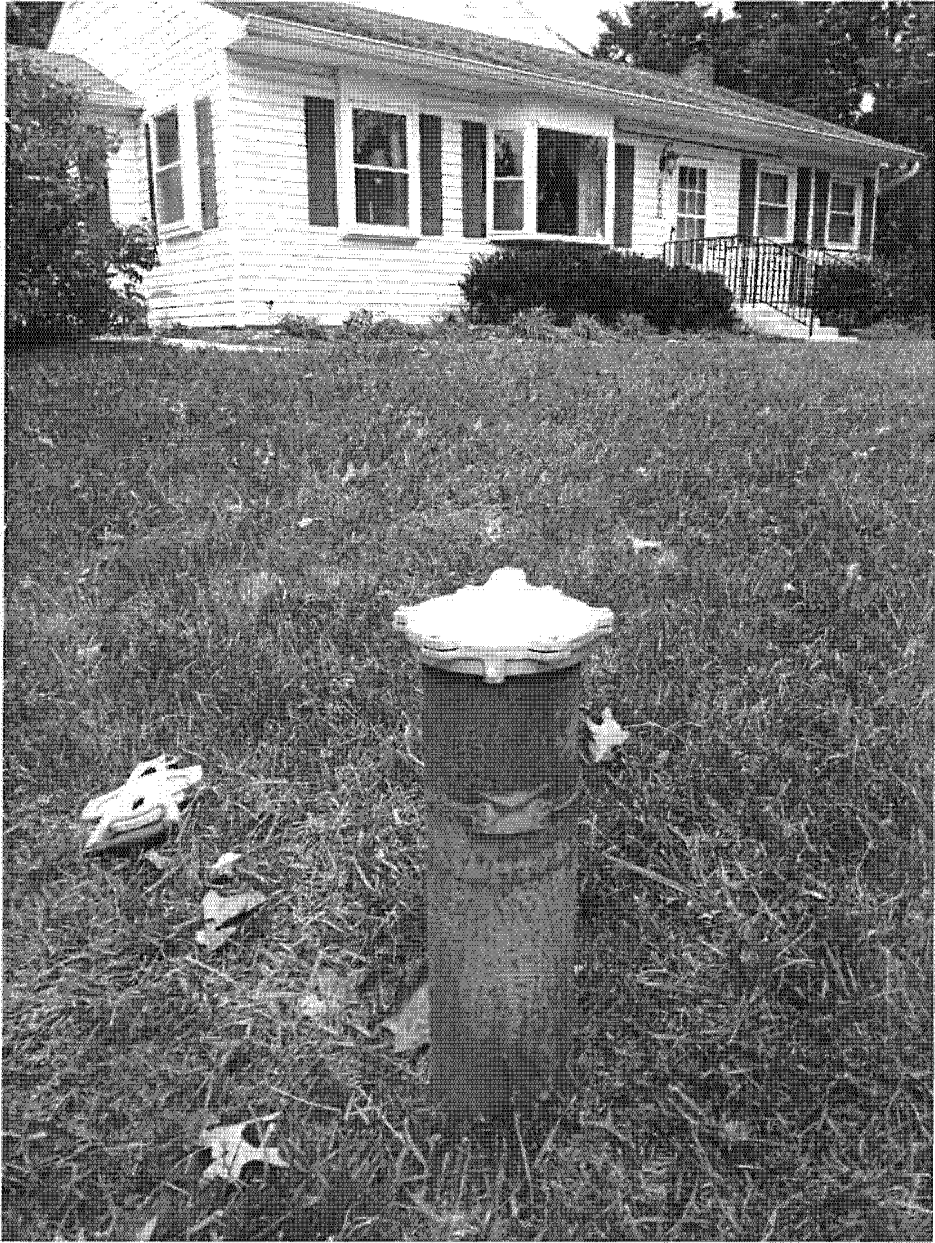
The two piece well cap is secured.
